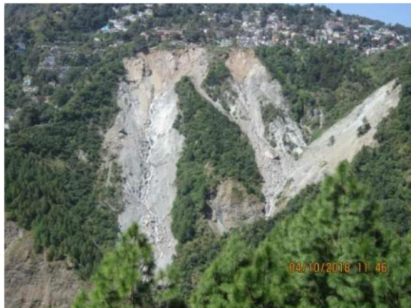
Photograph-1 A view of the Baliyanala Landslide (Source: DMMC, 2018)
