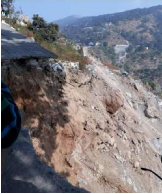
Photograph-2 Damaged slope and broken road
