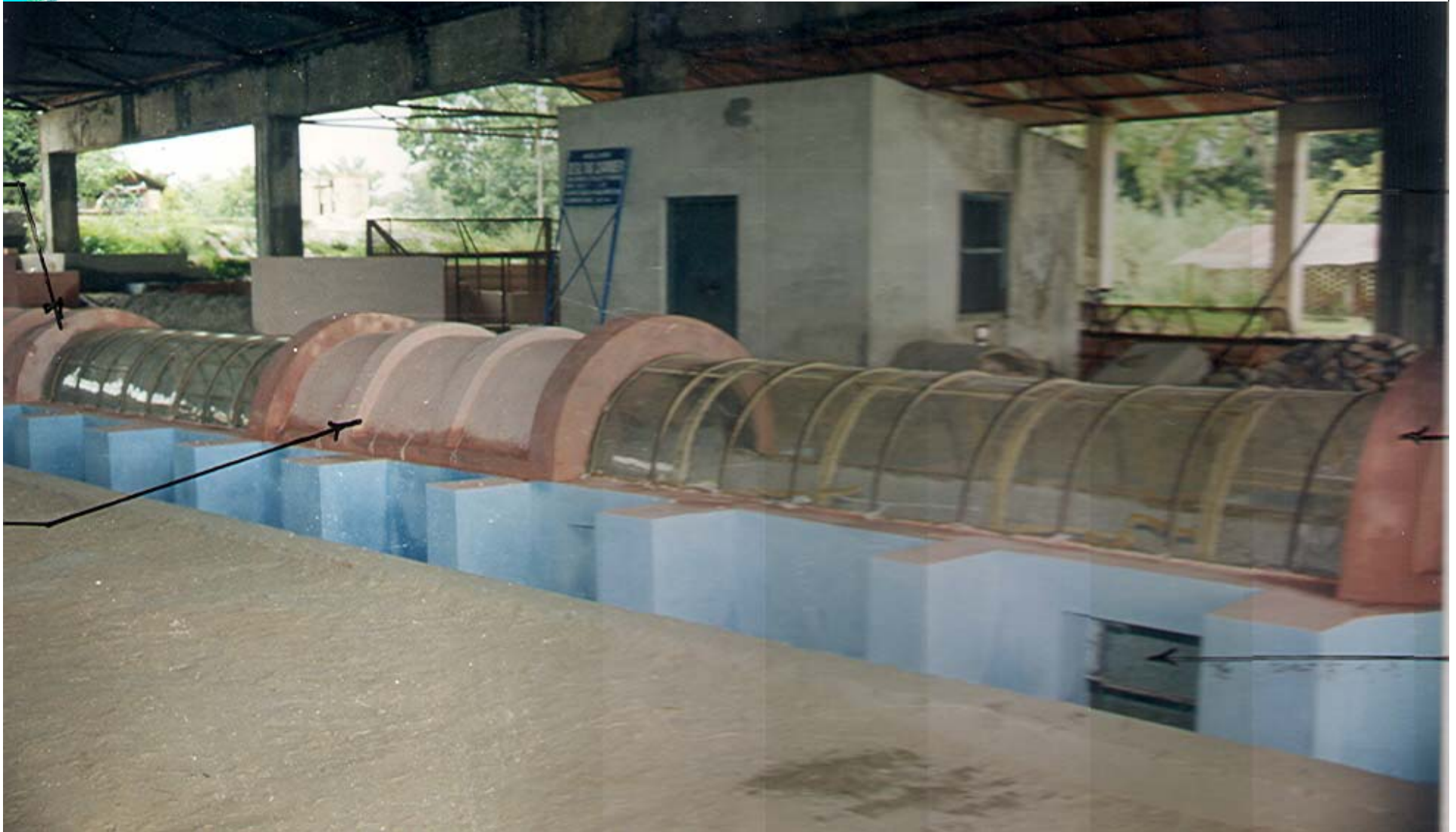
Desilting Chamber of Bhilangana Hydroelectric Project
